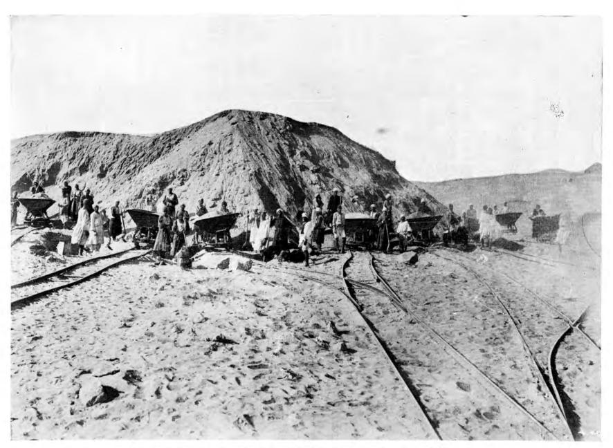
A view of part of our field of work at the beginning of the fifth season. Notice the method of laying the rails, which allows eight decauville cars to be in use, with a resulting economy of time.
